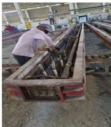
Fig 2: Placement of Reinforcement
