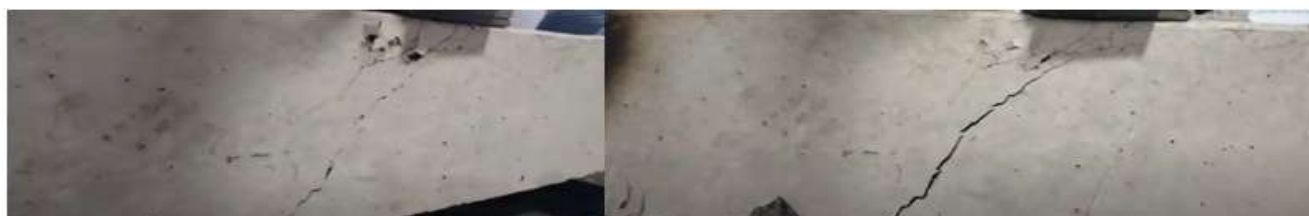
Fig 14: Failure moment at Rail seat - shear failure – Normal Concrete Sleeper
