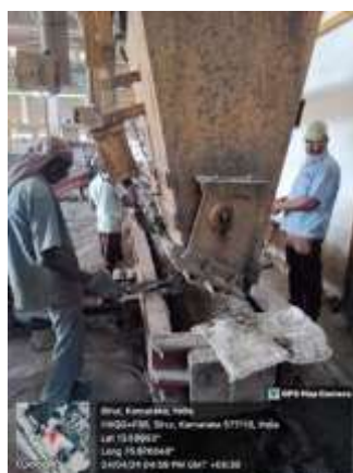
Fig 4: Casting Process of Sleeper
