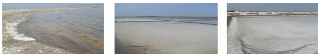
(1) Reservoir Pond (2) Evaporation Pond (3) Crystallization Pond
