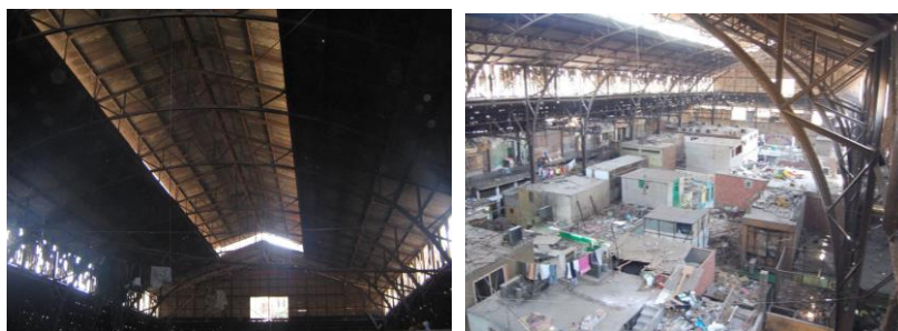
Fig. 13. Market's Steel Structure is in good condition. Source, Researcher
