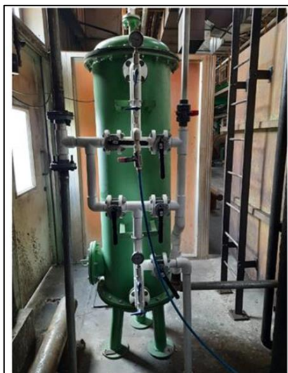
Figure 1: Sand and Pebble Filter
