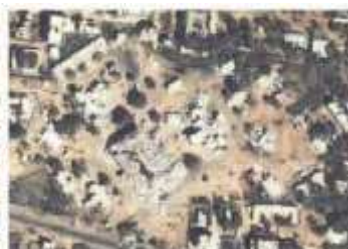
FIGURE 2. Collapse of a few buildings, in the modern side of the city
