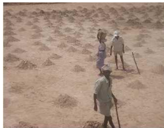
Figure 2: Scraping the bottom of pond (using man power)
