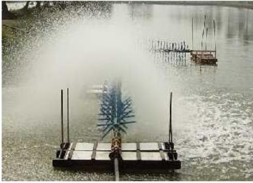
Figure 11: DO were enriched on the water surface using long arm aerators
